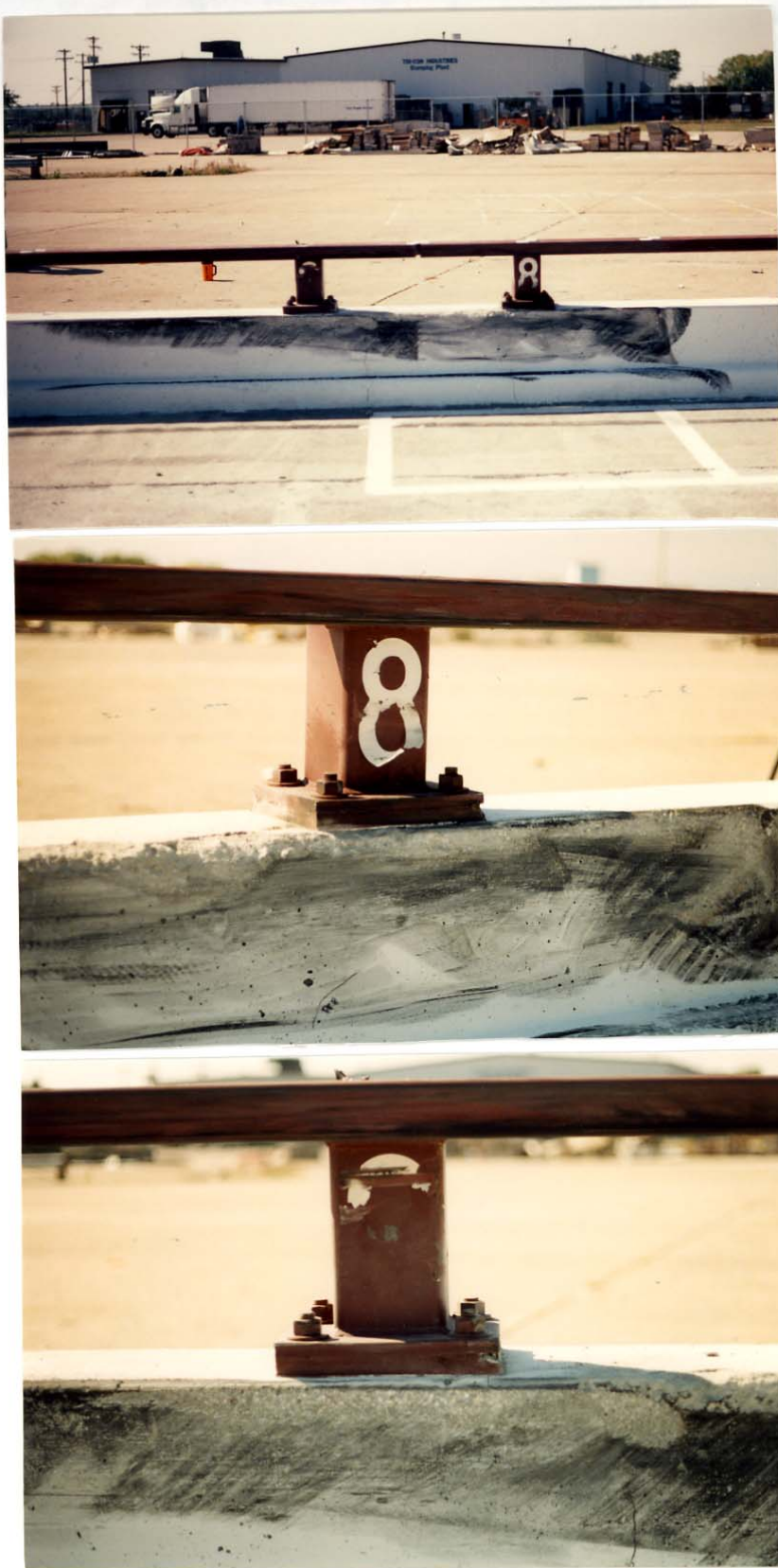
Figure 21. Bridge Rail Damage, Test MN-2.
