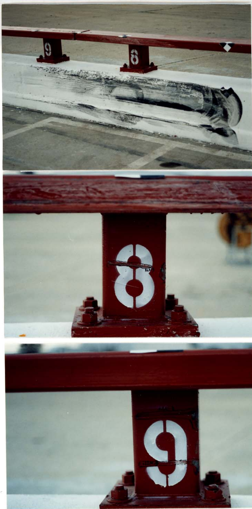
Figure 30. Bridge Rail Damage, Test MN-4.
