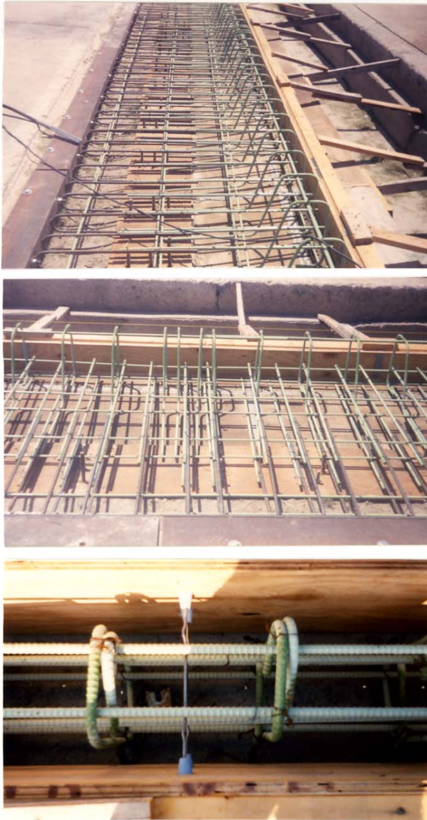
Figure 4. Reinforcement layout for bridge deck and parapet.
