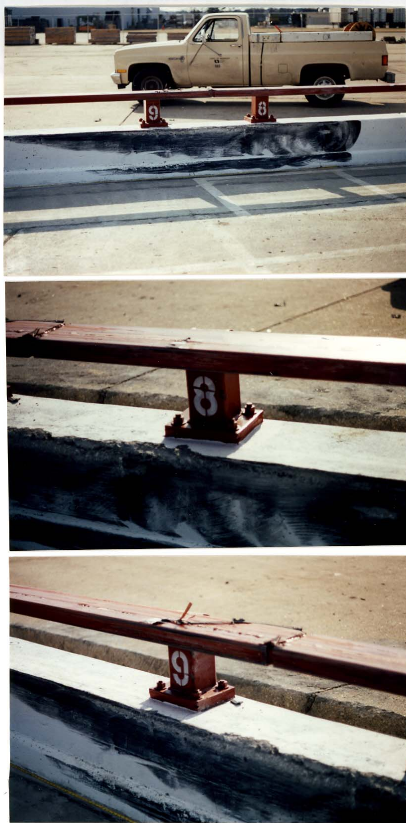
Figure 26. Bridge Rail Damage, Test MN-3.
