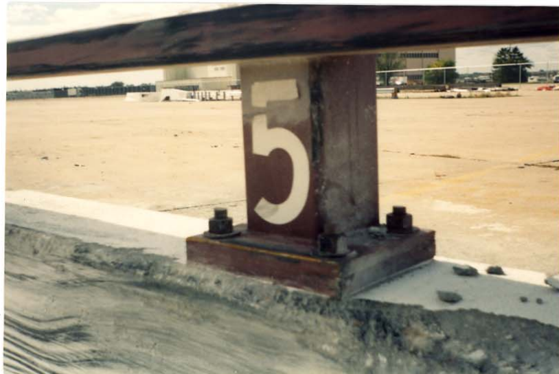
Figure 15. Bridge Rail Damage, Test MN-1.
