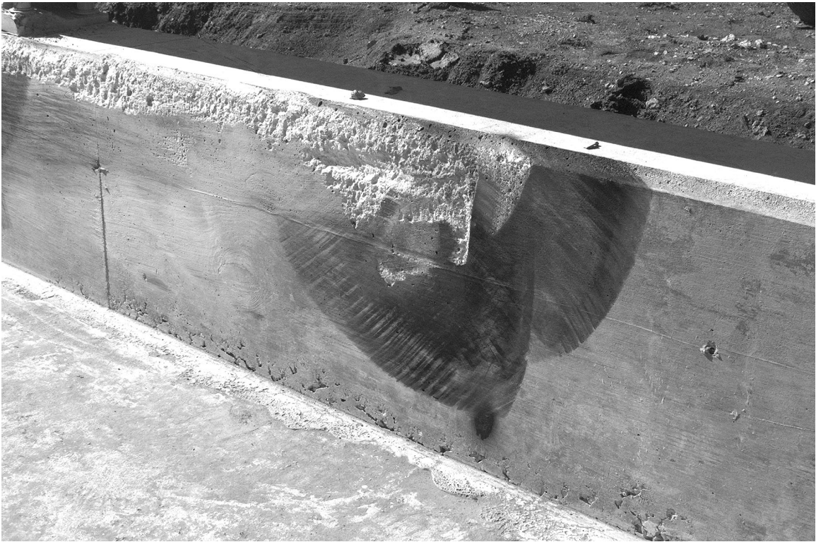
Figure 7. Installation after Test 418049-7.
