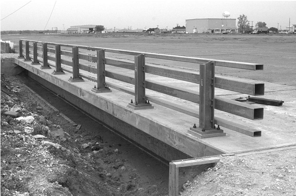
Figure 4. New York Four-Rail Curbless Bridge Railing Installation.
