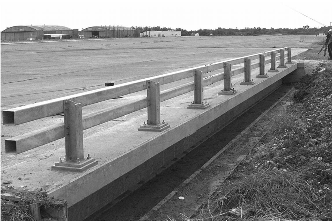
Figure 2. New York Two-Rail Curbless Bridge Railing Installation.
