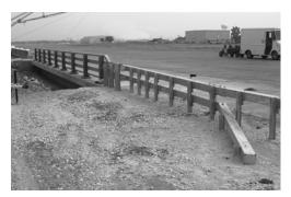
apron was broken off and sufficient reinforcing bars were added to join to the simulated bridge deck. A 21.98 m section of the New York Two-Rail and Four-Rail Curbless Bridge Railing was installed on the deck. Adjacent to the deck, the New York Box-Beam transition was installed in *NCHRP Report 350* standard soil. Further details of the three installations are presented in Chapter III.
