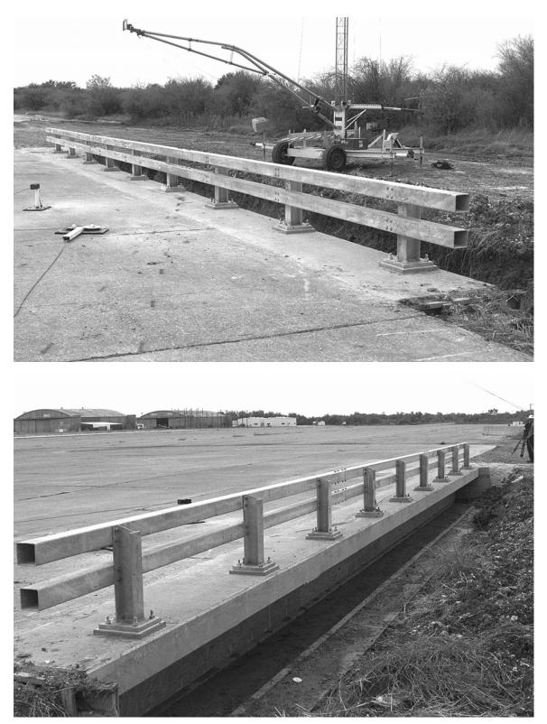
Figure 2. New York Two-Rail Curbless Bridge Railing Installation.
