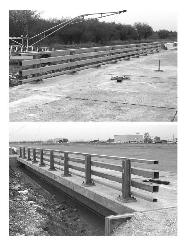
Figure 4. New York Four-Rail Curbless Bridge Railing Installation.
