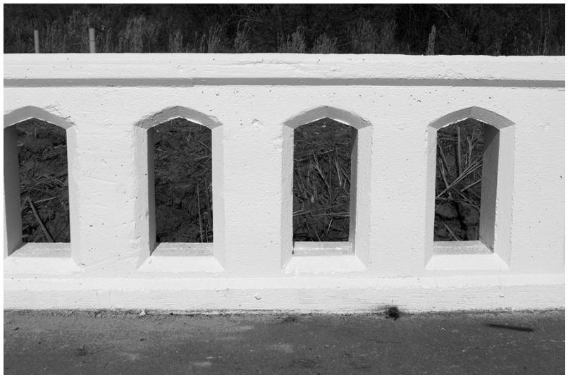
Figure 3. Texas Type T411 Bridge Railing Installation before Test 418048-1
