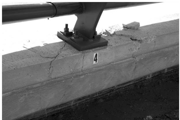
Figure 23. Installation after Test 442882-3.
