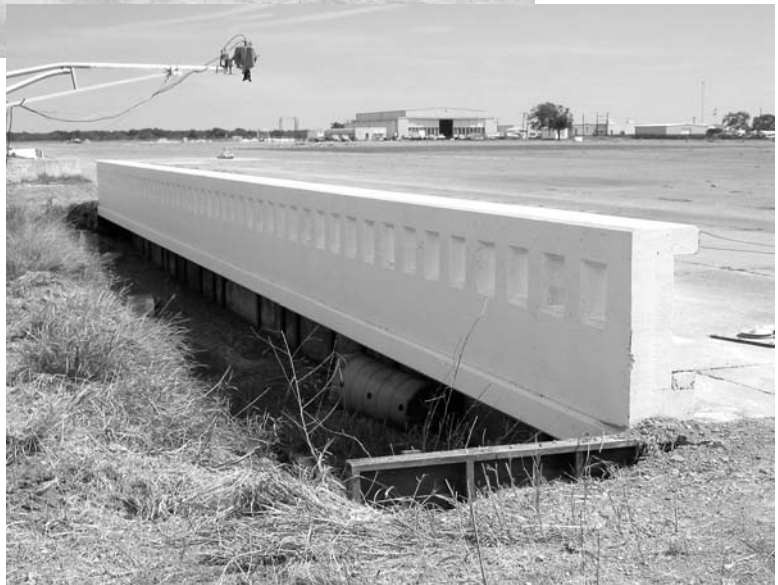
Figure 2. TxDOT F411 Bridge Rail before Test No. 421324-3.
