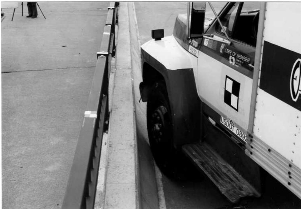
Figure 33. Impact Location, Test MNPD-2
