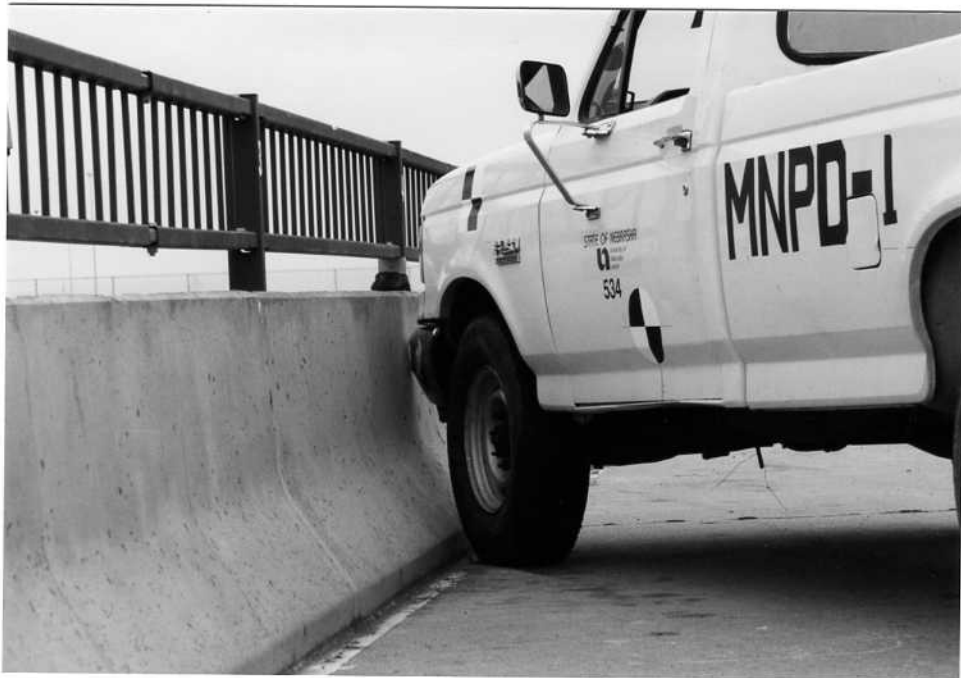
Figure 23. Impact Location, Test MNPD-1
