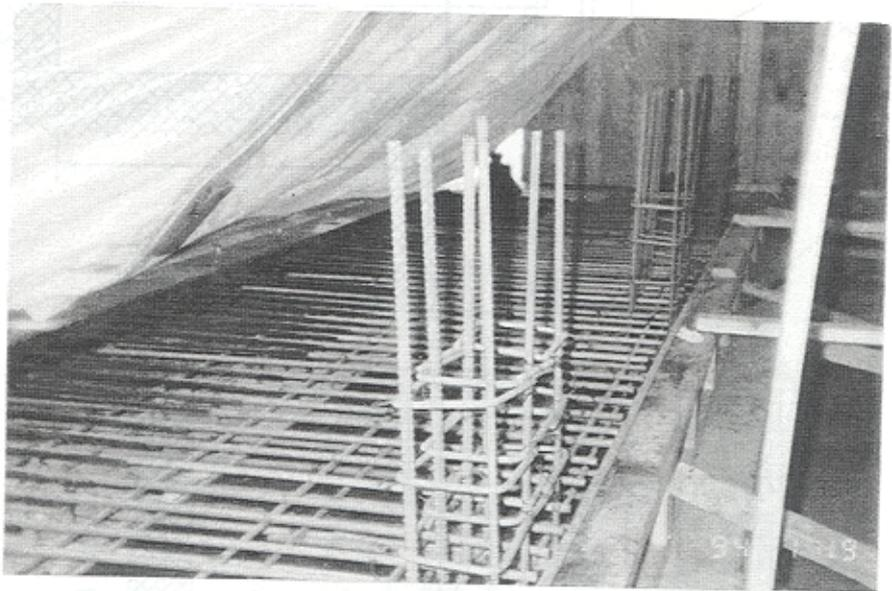
FIGURE 5. Reinforcement Layout for Bridge Deck
