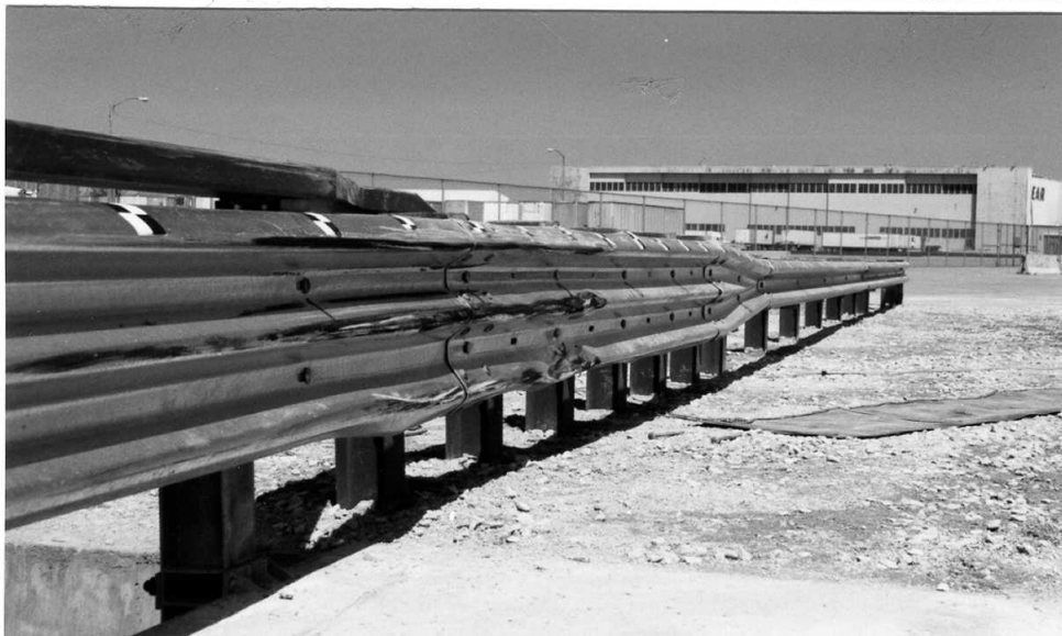
Figure 172. Barrier Damage, Test STTR-3
