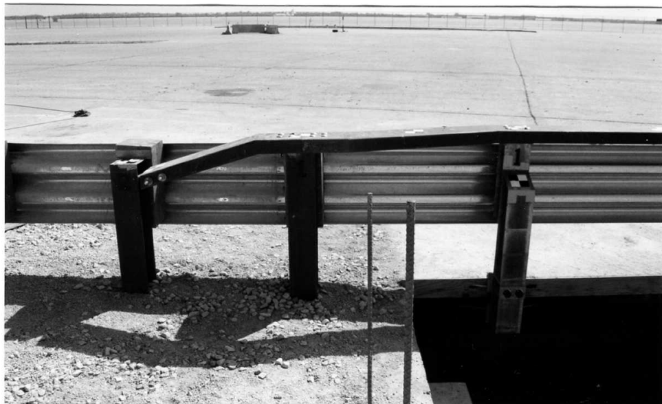
Figure 131. Connection to Steel Bridge Railing System
