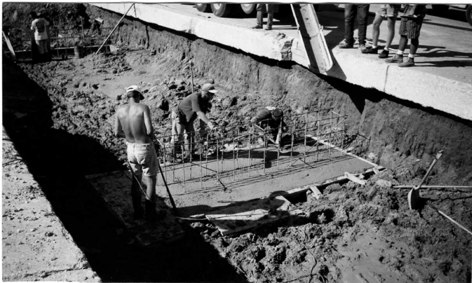
Figure 5. Bridge Substructure Construction
