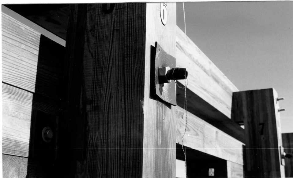
Figure 88. Steel Plate Deformations at Post No. 6, Test TRBR-2
