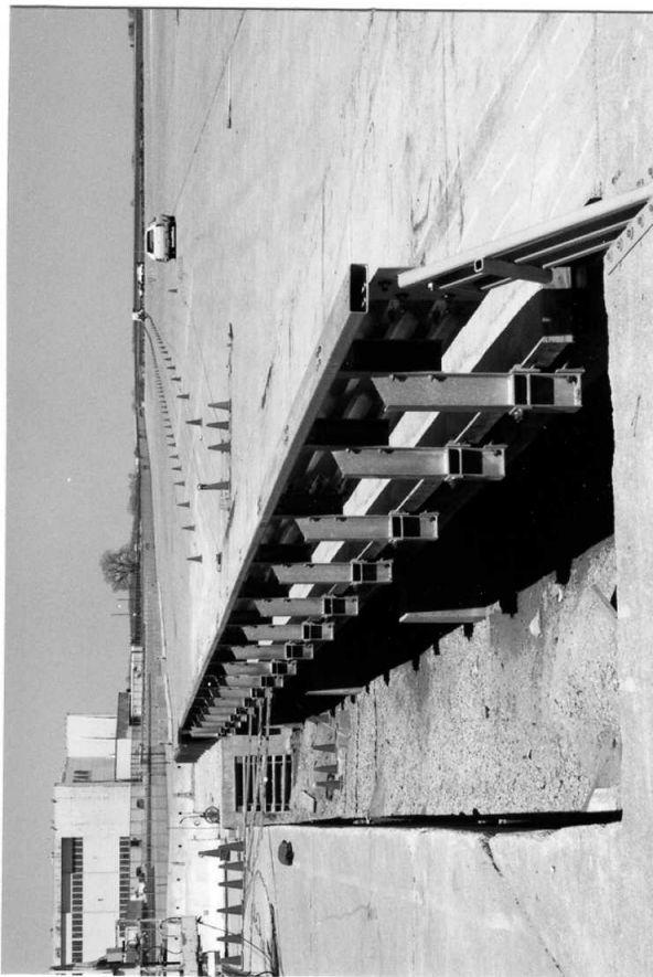
Figure 116. Steel Bridge Railing System
