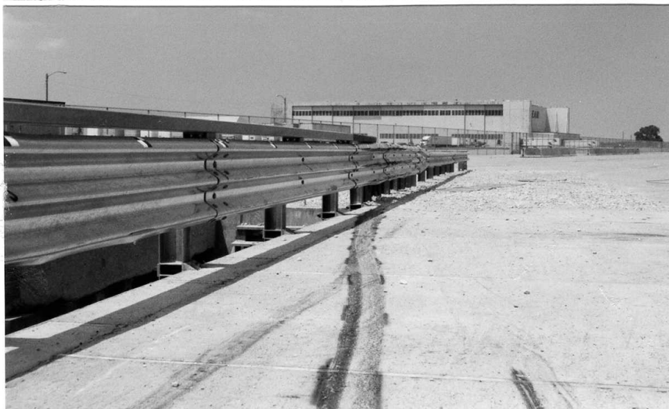
Figure 186. Barrier Damage, Test STTR-4
