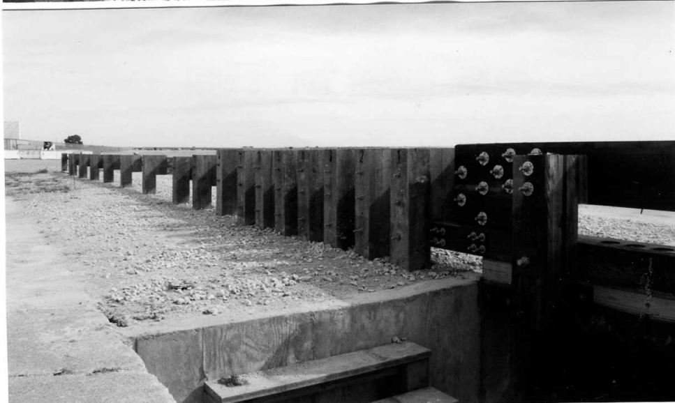
Figure 56. Approach Guardrail Transition - Back View
