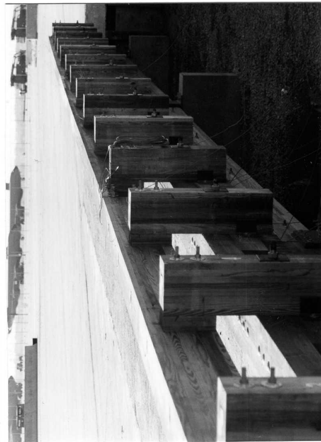
Figure 46. Wood Bridge Railing System
