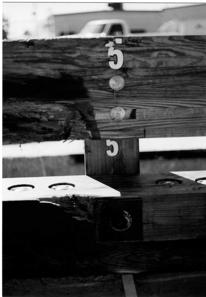
Figure 87. Barrier Damage, Test TRBR-2
