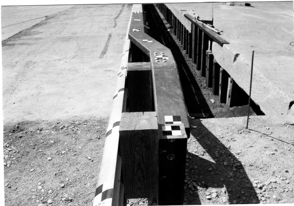
Figure 130. Approach Guardrail Transition - Parallel View
