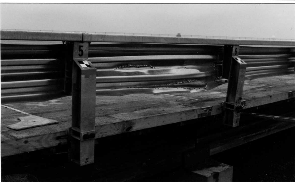
Figure 146. Barrier Damage, Test STTR-1
