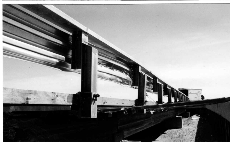
Figure 158. Barrier Damage, Test STTR-2
