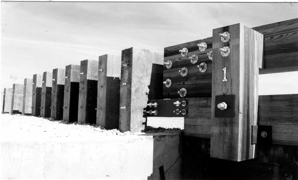
Figure 58. Connection to Wood Bridge Railing System
