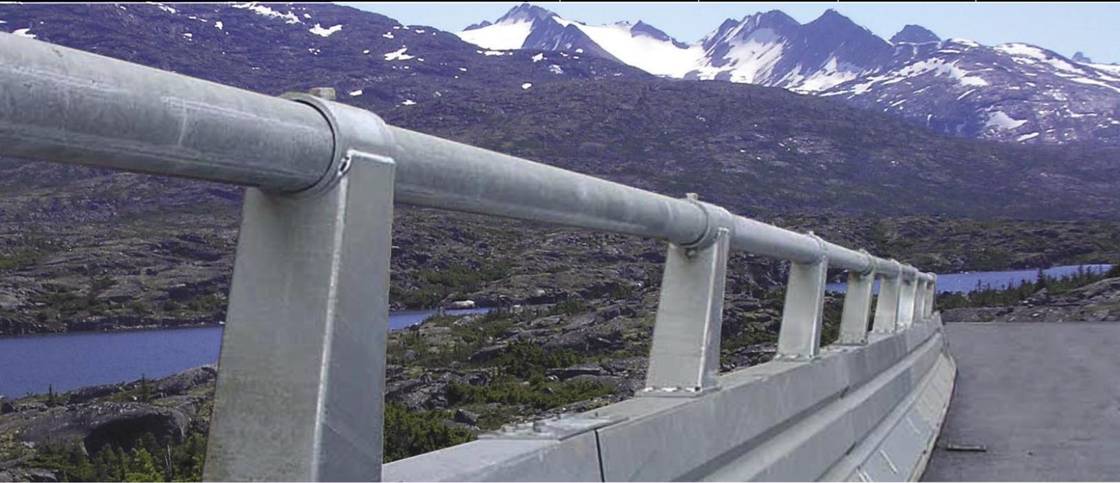
MDS bridge railing system can be utilized for new bridge construction projects or on rehabilitation bridge projects. The unique energy dissipating slip base connectors, anchored with mechanical or chemical anchors, may reduce deck damage by minimizing the force from impacts transmitted to bridge deck.
