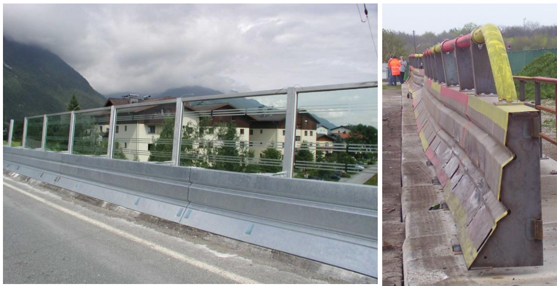
Figure 1. Photographs of the MDS-4 barrier with noise-wall installed (left) and a post-collision photograph of the MDS-5 barrier without the noise wall installed
