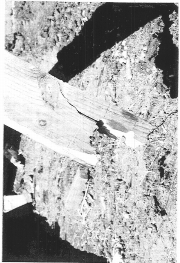
Figure 34. Typical Bridge Rail and Post Damage, Test LVBR-2
