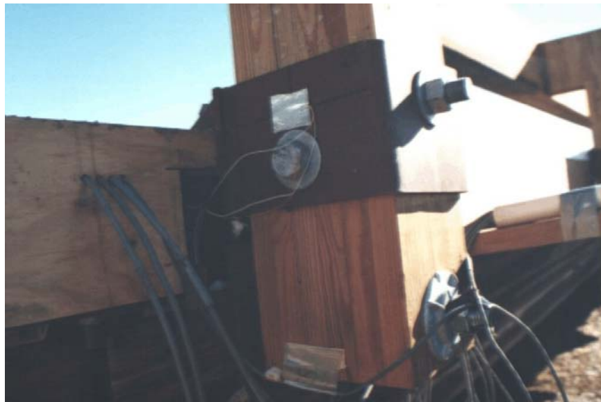
Figure 27. Typical Strain Gauge Locations, Test WRBP-1
