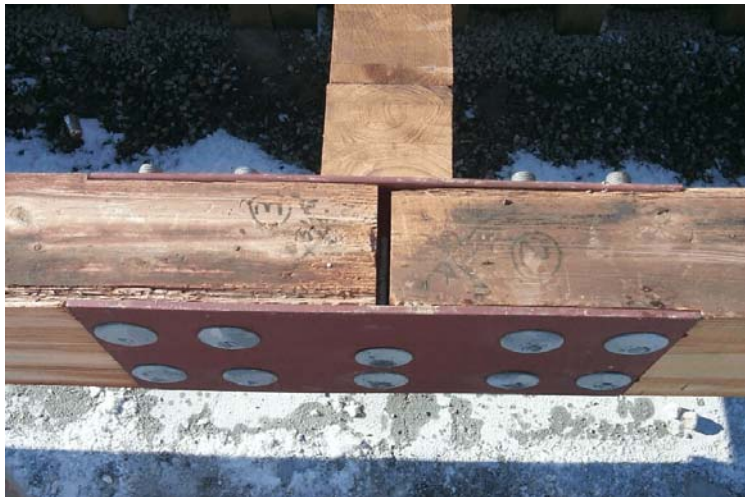
Figure 87. Wood Bridge Railing System - Rail Splices
