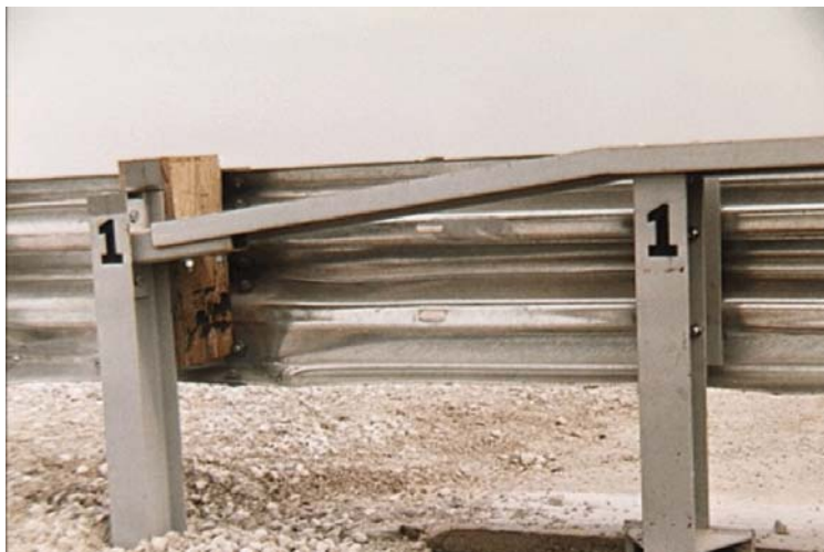
Figure 77. Barrier Damage, Test STCR-2
