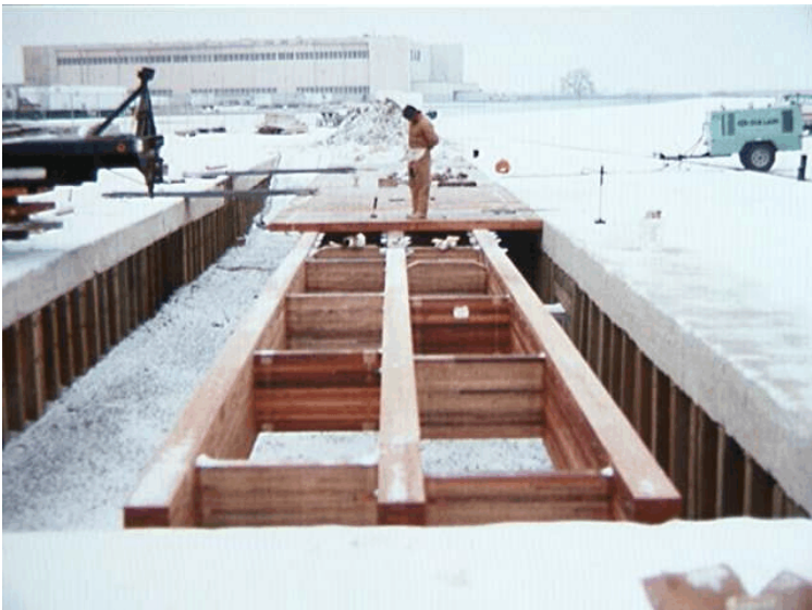
Figure 8. Bridge Superstructure Construction
