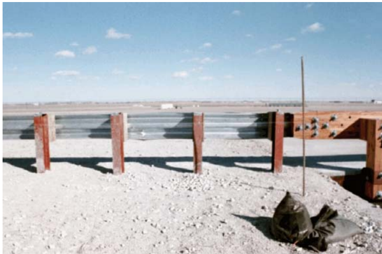
Figure 124. Barrier Damage, Test WRBP-2
