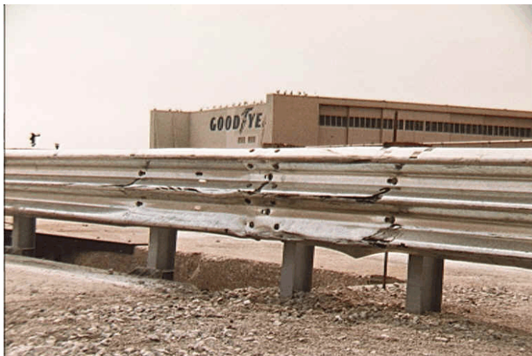
Figure 76. Barrier Damage, Test STCR-2
