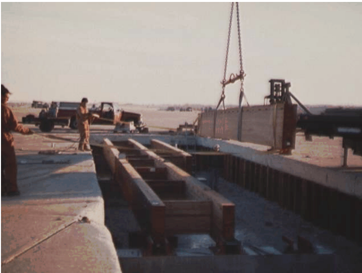
Figure 7. Bridge Superstructure Construction
