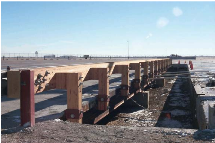
Figure 84. Wood Bridge Railing System
