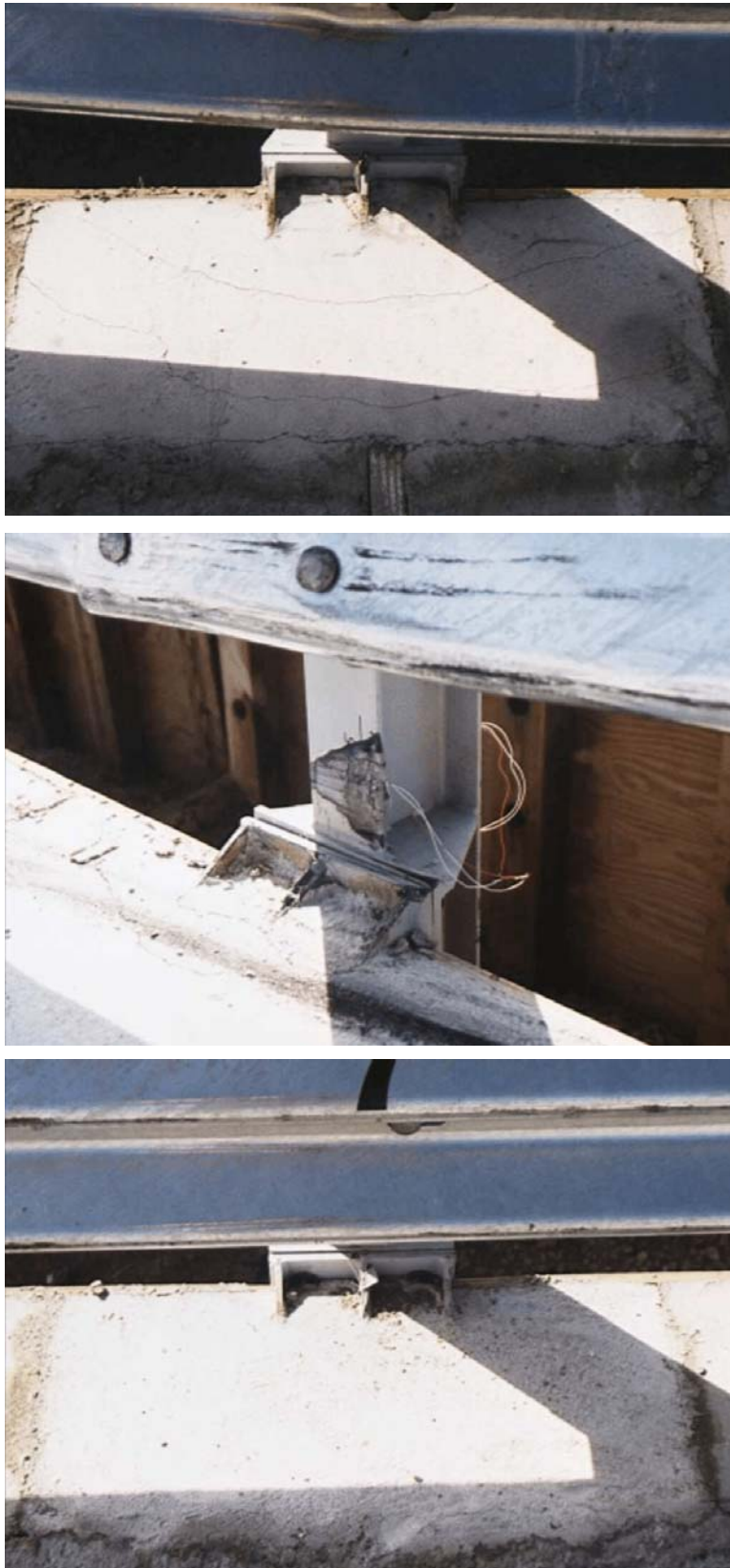
Figure 63. Cracking in Portland Cement Concrete Overlay, Test STCR-1
