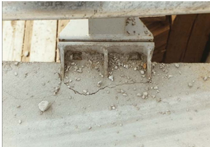
Figure 79. Bridge Post No. 1 Damage, Test STCR-2
