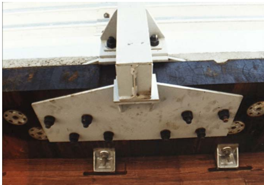
Figure 30. Steel Bridge Railing System - Bridge Posts
