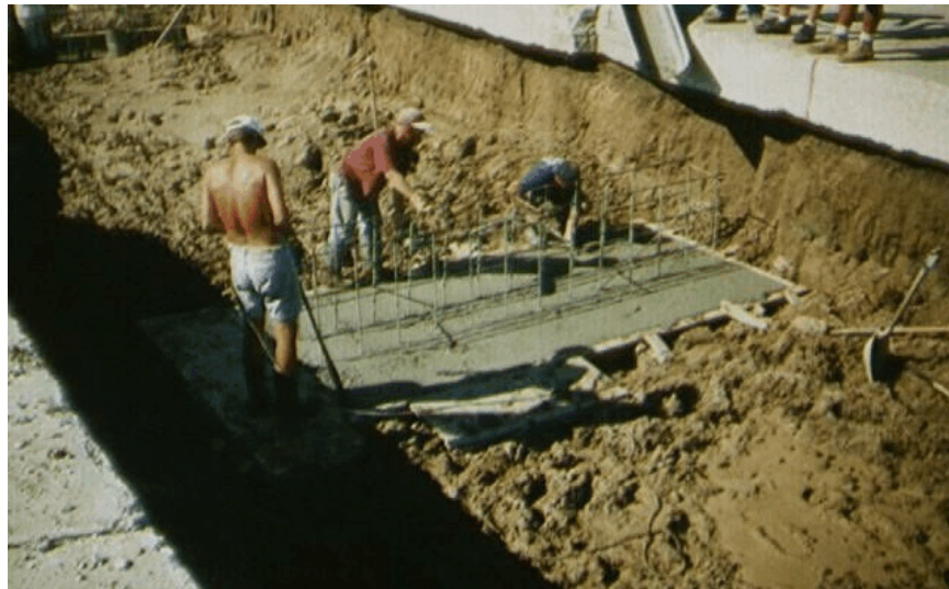
Figure 5. Bridge Substructure Construction
