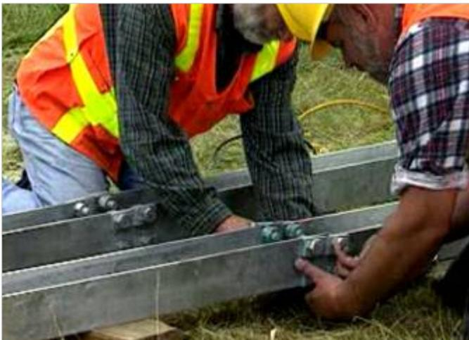
7. For hinge assembly, place the upper and lower post sections together on a flat level surface. Place the hinge plates on the outer surface of the post and install and tighten bolts.
