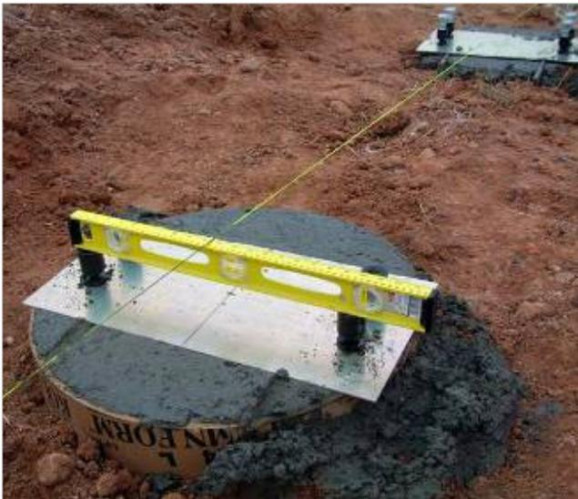
4. It is important to square and level the anchors that are attached to the template.
