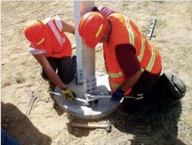
**12. Tighten the special bolts while holding the coupling by the upper wrench flats.**
