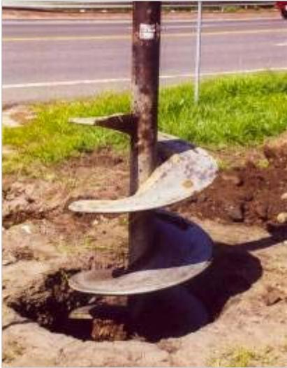
3. Auger the hole for the foundation and position reinforcing.
