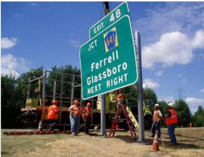
**13. After all of the posts are secured in place, attach the sign panel assembly to the post in accordance with the sign manufacturer's recommendations.**
