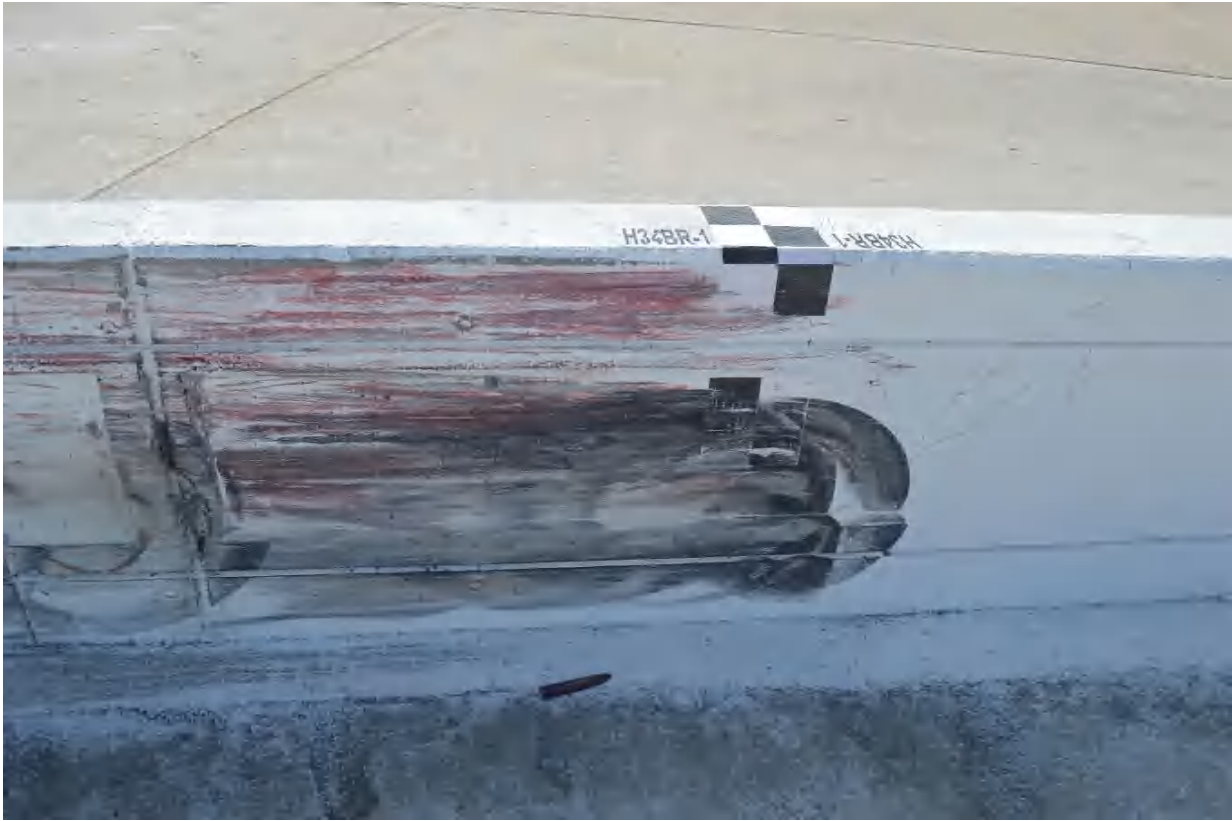
Figure 36. Traffic-Side System Damage, Test No. H34BR-1
